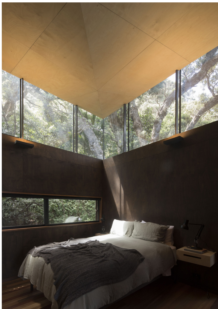
Above The main bedroom is contained within ply walls stained the same tone of pōhutukawa branches. The fold in the ceiling required detailed 3D modelling to resolve its structure.
