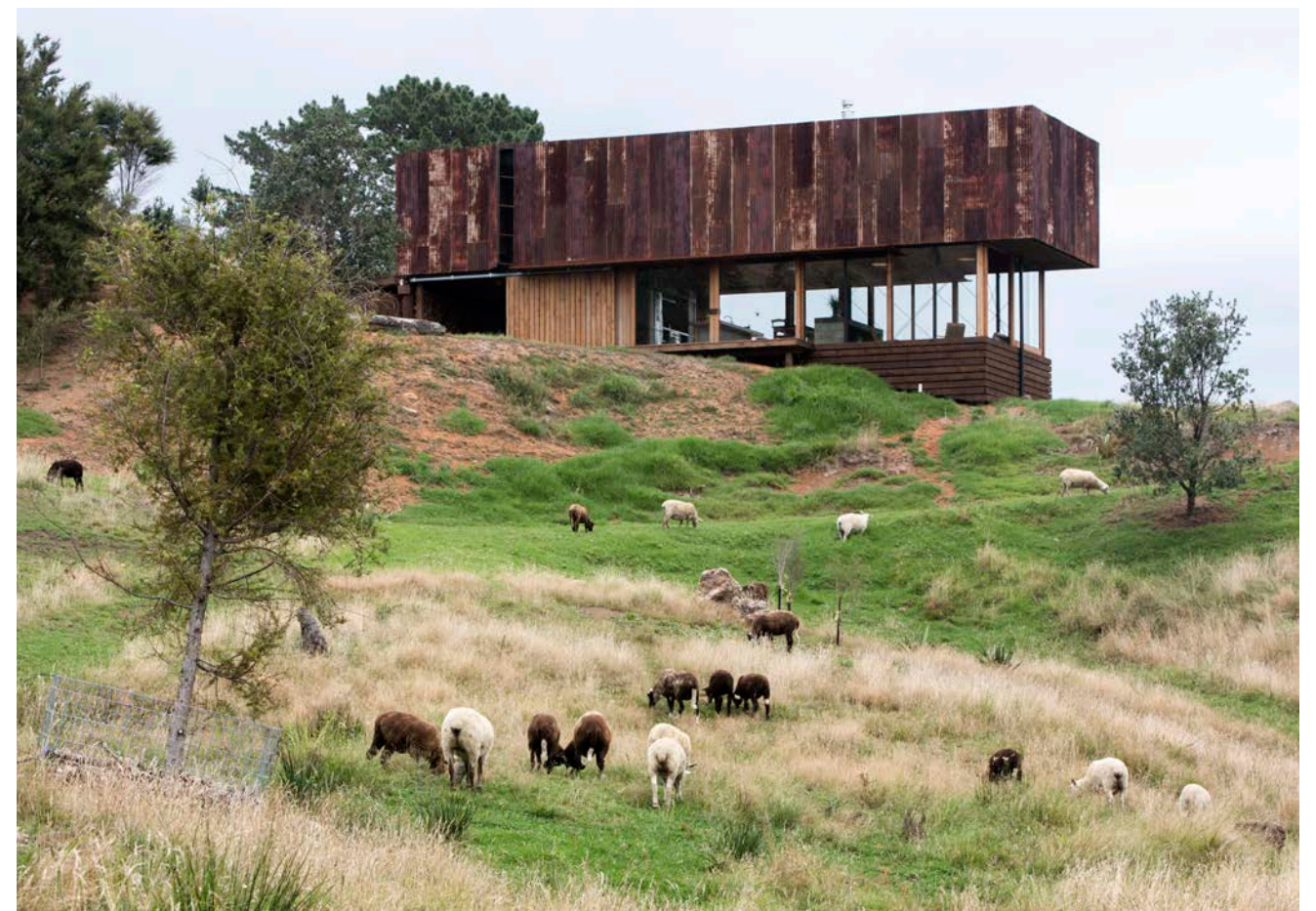
The resolute, blunt-edged form is a deliberate departure from Herbst Architects' previous work and an “active disruption” of their customary approach to designing homes – it could be described as agrarian brutalism. “We just felt the need to come at things from a slightly different angle,” says Lance Herbst.
